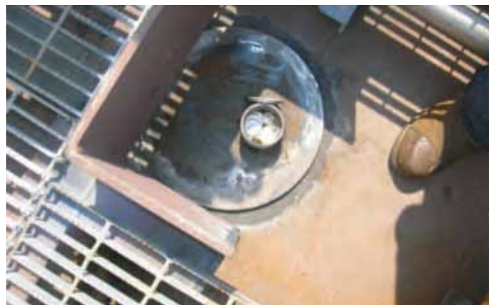
The coins in place at the mast foundation
